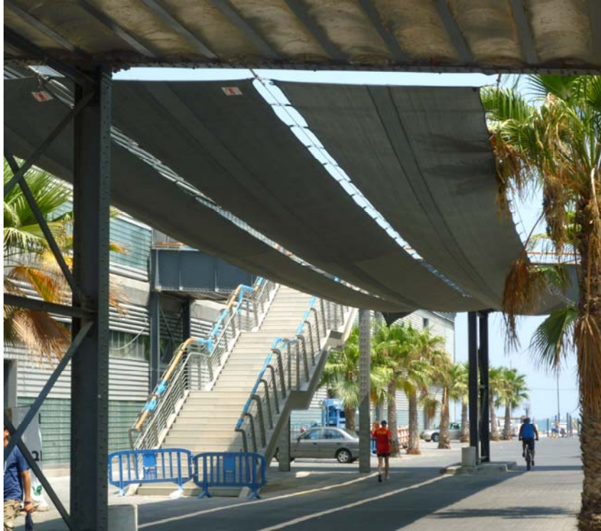
Fig. 19: Tarpaulins stretched across a street as a local measure to mitigate human heat stress in a Mediterranean coastal city (Jaffa, Israel)
